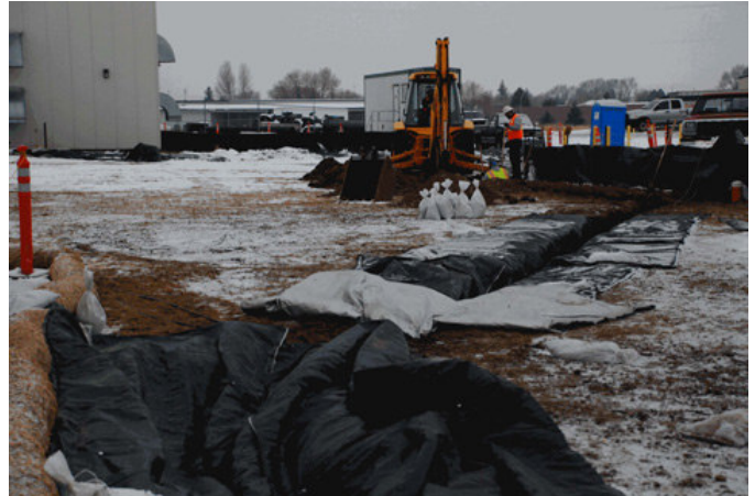
Underground utilities were installed during site preparation work in March 2010.
